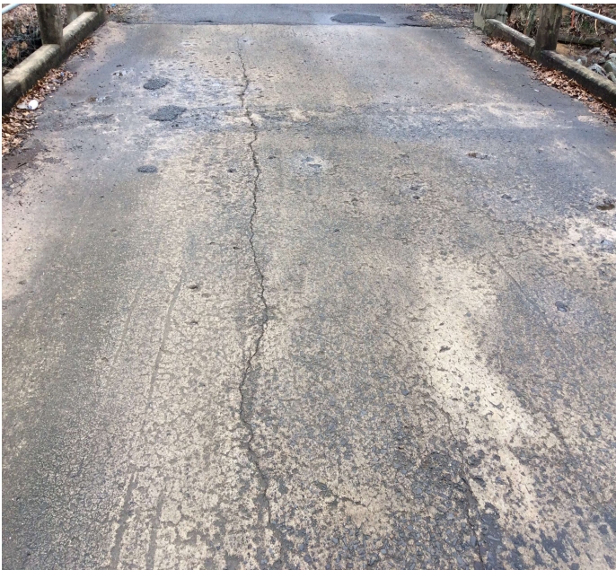
PHOTO 1 Description Deck crack.
