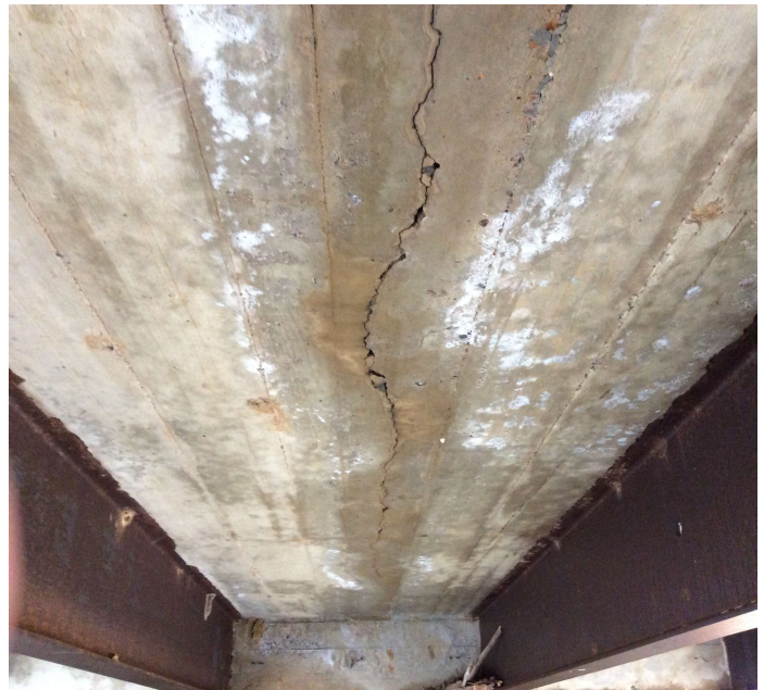
PHOTO 2 Description Deck soffit crack. Bay 2.
