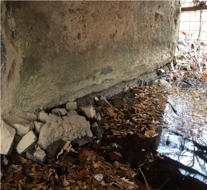
PHOTO 3 Description West abutment. Soft deteriorated concrete.
